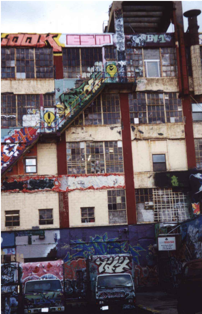
Building in Queens Photo: Holly Arden
